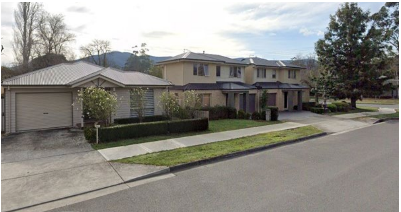
Figure 42. A recent example of a two-storey attached townhouse development in Yarra Junction, as it sits beside lower-rise development in the streetscape
